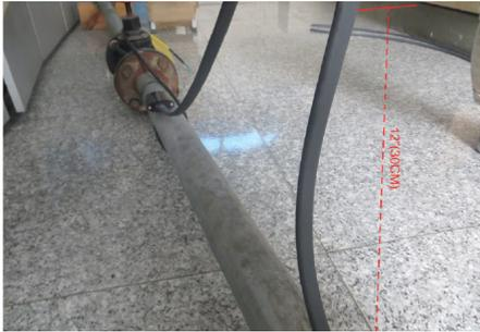
2- Insert the Pressure Seal End first and then the grommet for each cable.
