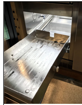
Fig. 1 Access the water reservoir
