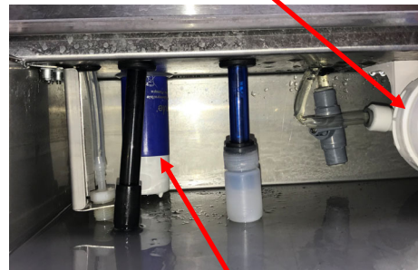
Water circulation pump; white filter cap at bottom
