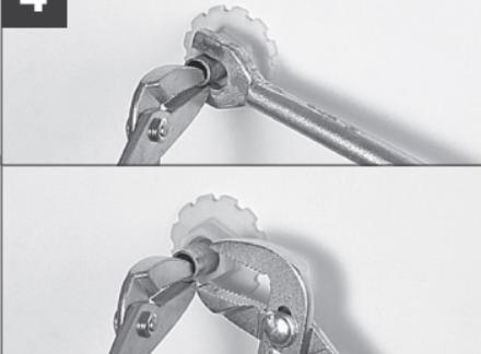
Cut excess copper stub out off leaving exactly 1½" to finished wall, then push Shower WallNut over remaining copper.
