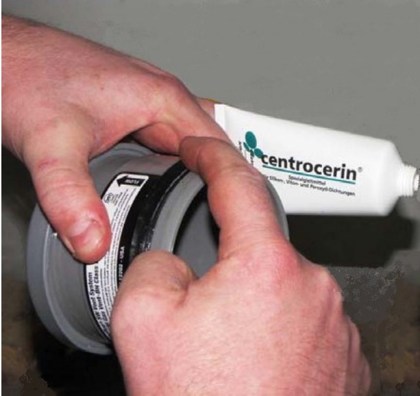
Applying Lubricant to Gasket
