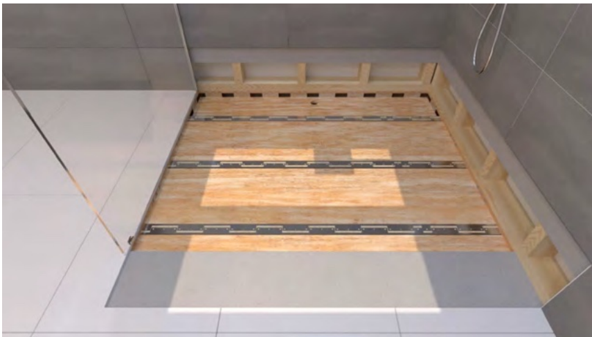
3. RECESS THE SUBFLOOR
