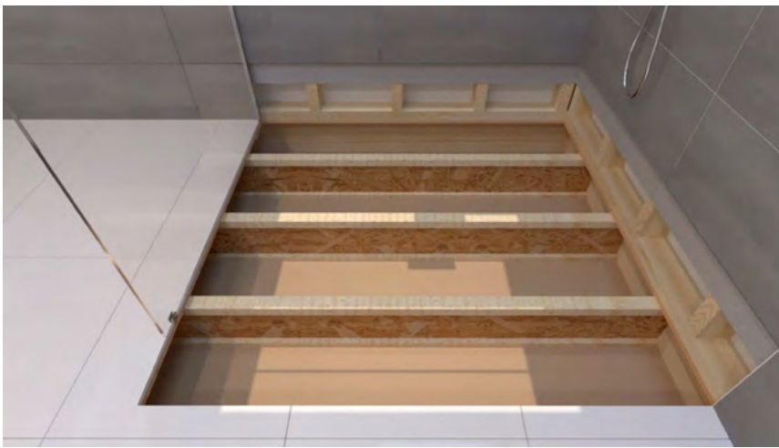
1. EXPOSE THE JOISTS
