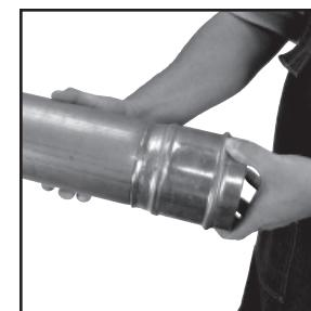
9. Allow the pressing cycle to complete. Then remove the pressing tool and adapter jaw from the pressing chain. Remove the pressing chain from the fitting.
