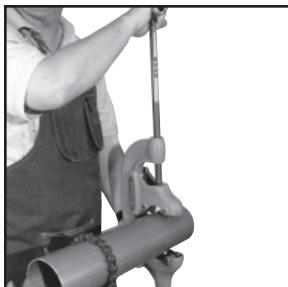
1. Select clean, undamaged copper tube and cut square with a tube cutter to the desired length.
