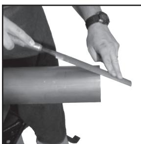
3. Deburr the tube outside diameter using a half-round file to prevent damage to the EPDM seal. Clean the tube end of all contamination, oils, shavings and oxidation. A smooth transition chamfer is recommended to ease tube insertion past the seal.
