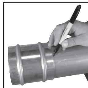
5. Mark the proper insertion depth on the tube with a permanent marker *prior* to insertion, based on insertion depth chart. Insert the tube into the fitting end using a twisting motion. Make sure that the tube is fully inserted. **If tube is not inserted to the proper depth, an inadequate seal may result.**
