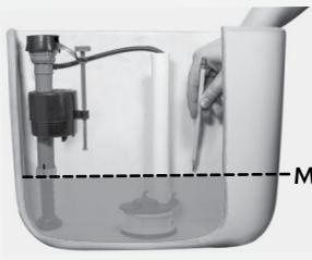
**c) Remove old flapper. Install new flapper. Attach chain to flush lever with minimal slack.**
