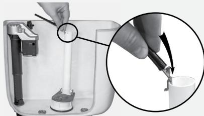
c) Attach other end of tube to refill adjuster. If tube kinks or is too long, trim prior to attaching.
