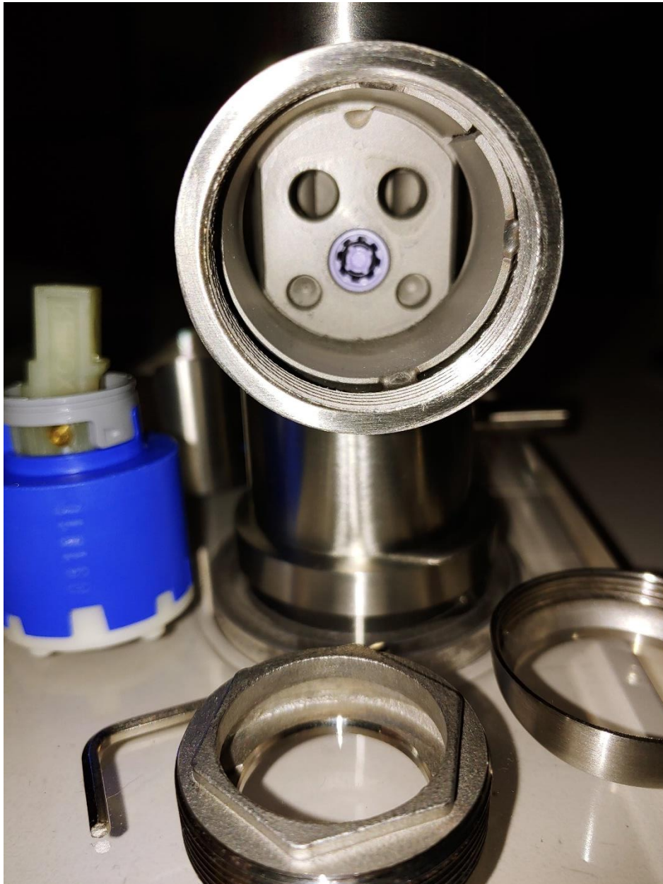
This is what the faucet looks like with the cartridge removed
