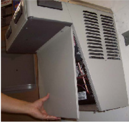
Remove Front Panel
