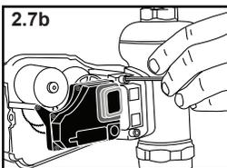
2.7 Place the Electronic Flush Device on to the flush valve handle (a). Make sure unit is pushed all the way on to the handle. Position unit as desired (rotate if needed), place mounting clamp over the handle and (b) tighten with Allen key.
