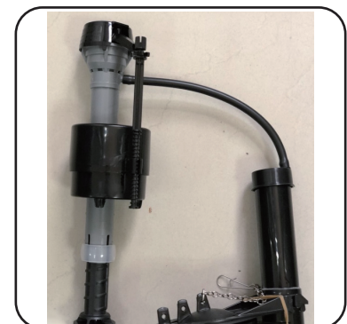
Correct set up of refill tube
