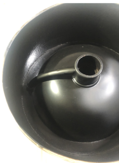
Overflow fitting close-up
