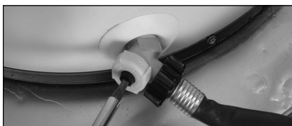
Figure 39 - Draining the water heater.
