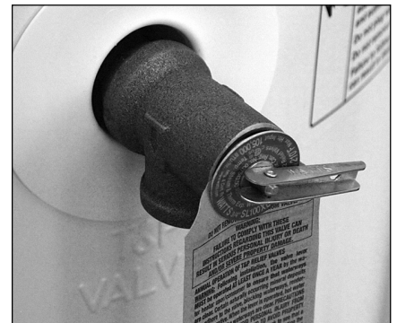
Figure 24 - Temperature and Pressure Relief Valve
