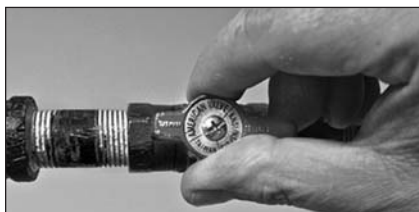
Figure 49 - Gas valve in “on” position.
