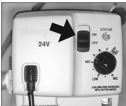
Figure 37 - Turn gas control/temperature knob OFF.
