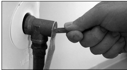
Figure 42 - T&P Relief Valve.
