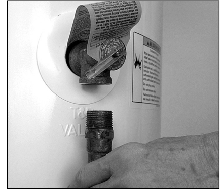
Figure 21 - Removing the T&P Relief Valve discharge pipe.
