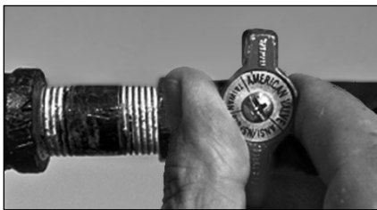
Figure 45 - Gas valve in "off" position.
