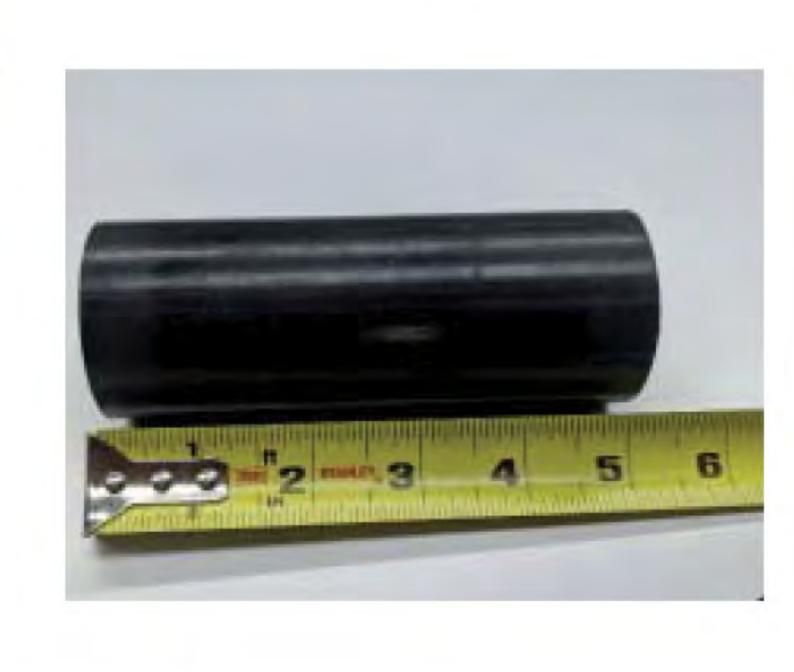
4. Apply ABS glue to the outside of the ABS 1 ½" pipe and to the inside of the P-trap.
