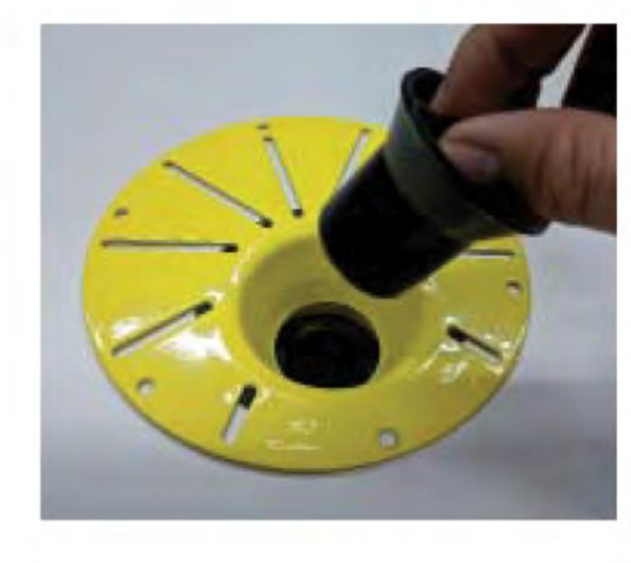
11. Apply provided lubricant inside black plastic tubing of the Drop-In Drain.
